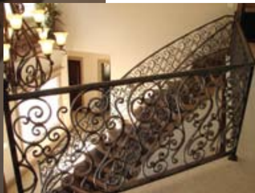
Hand forged scroll railing was created to match the ironwork on the front door. A radius (curved) staircase is challenging to fabricate.
